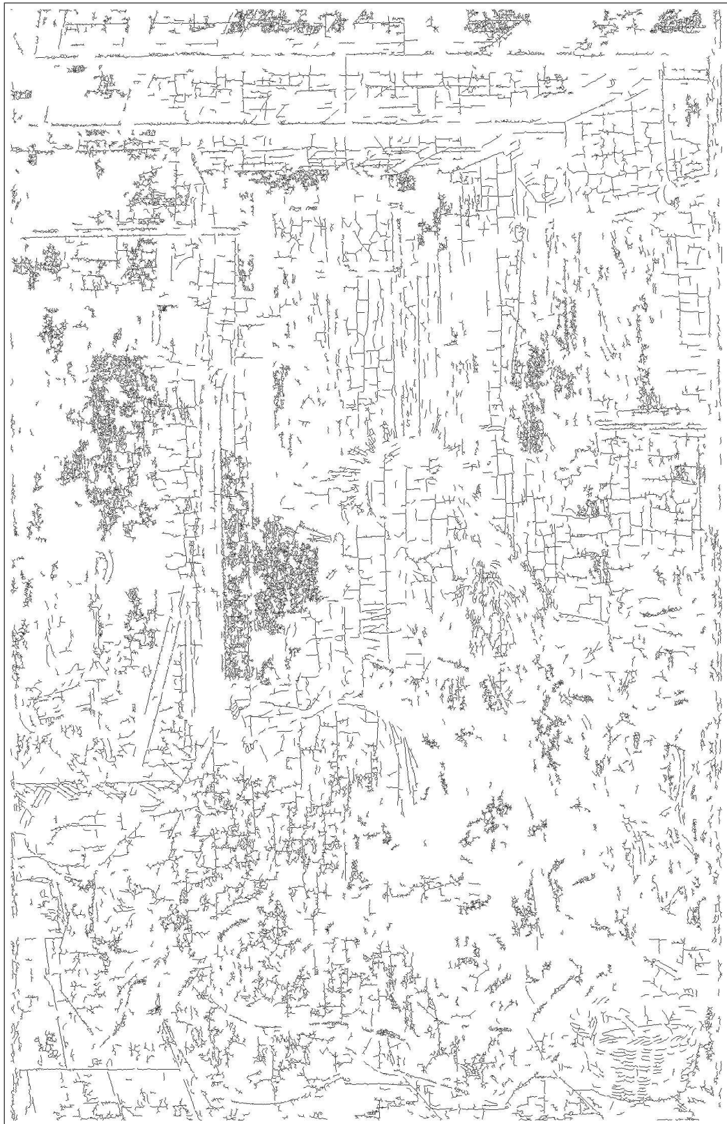
Figure A.4: Crack detected version of Figure A.3. Notice the edges and painting details such as brush stroke patterns are also detected due their crack-like characteristics. The process took 3 hours, 47 minutes and 50 seconds to complete.
